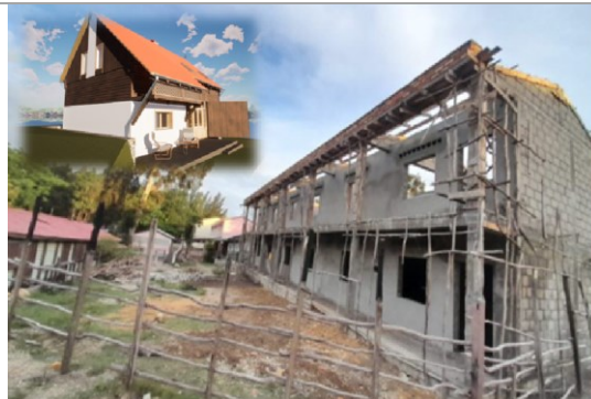
House renovation (insert showing final structure)
